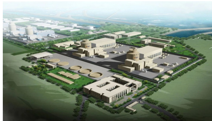
2*CAP1400 Shidaowan Units 1 & 2
