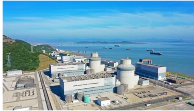
2*AP1000 Haiyang Units 1&2 (Finished)
