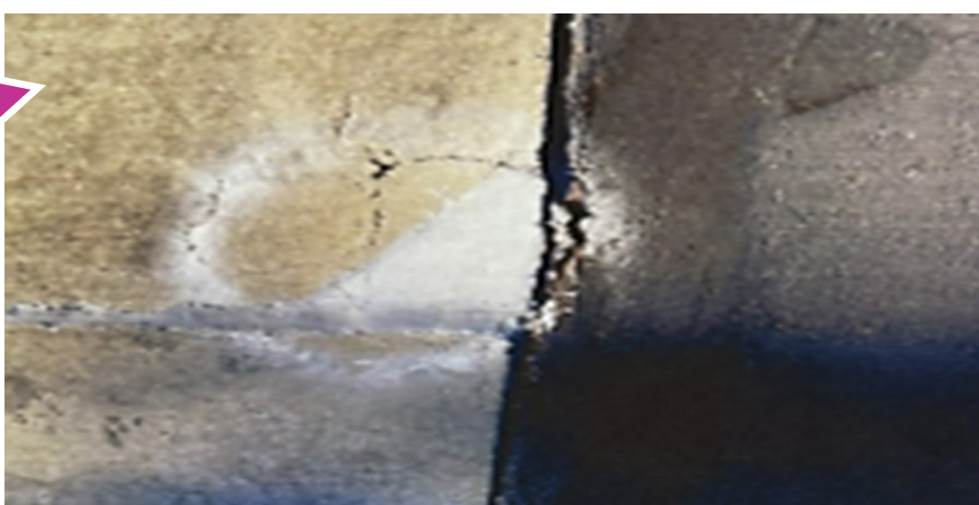
Figure 4. Concrete cracks
